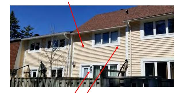
Installed new aluminum capping, new coach lights, new aluminum fascia and soffit
