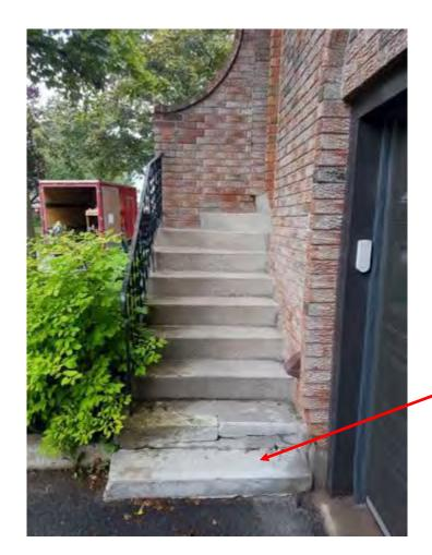
Cast iron railing replaced with aluminum railing
