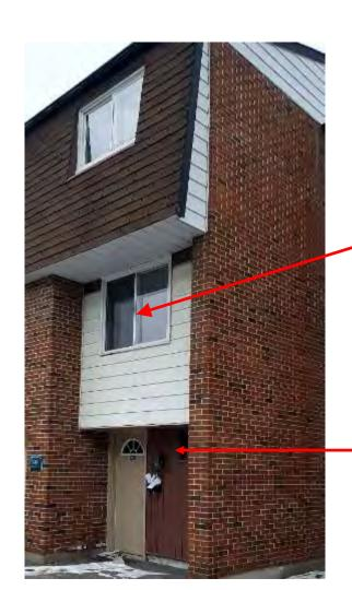
Replaced Mansard shingles with Enviroshake shingles
