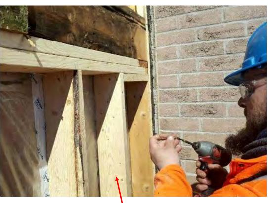
Replaced insulation, installed new framing members
