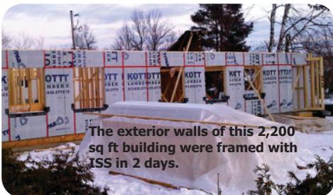
ISS from KOTT is available in precision-built 4'x8' sheets, and in thicknesses that deliver R-4 or R-5.6 thermal resistance values.
